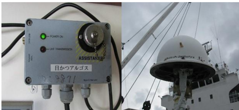
Figure 16 Argos MARGE unit with power light on and corresponding antenna
