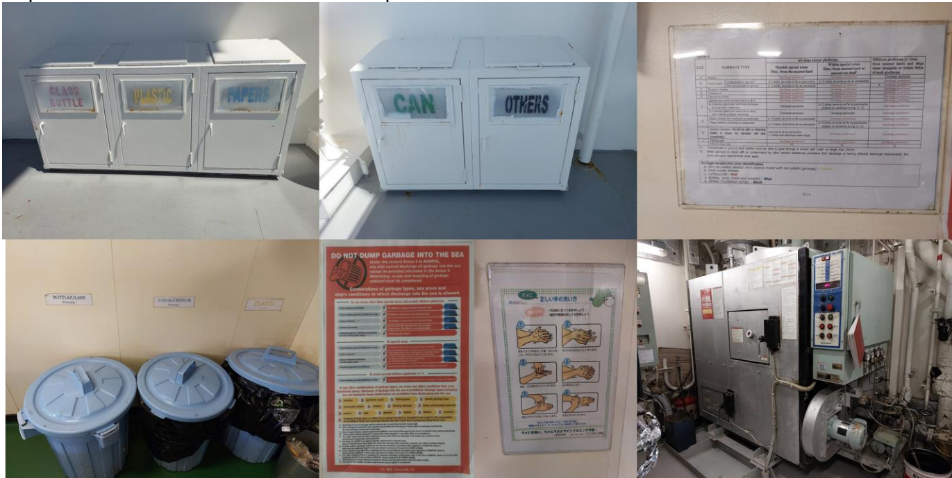
Figure 3 Waste disposal system onboard the CV
