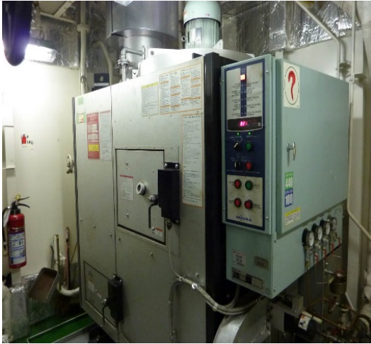
Figure 26 Engine room waste incinerator
