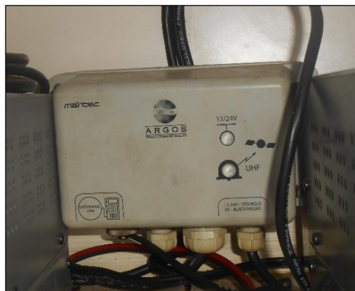
a) VMS unit, no power light was visible
