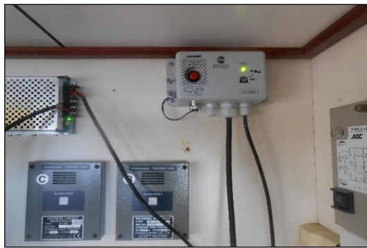
d) VMS after second inspection (
