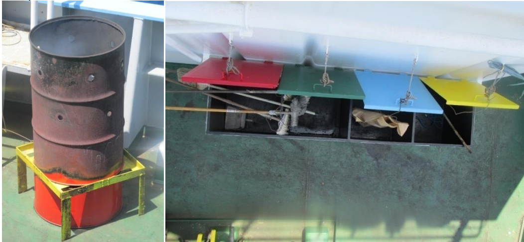
Figure 9 CV Incinerator (left) and waste disposal bin (right).
