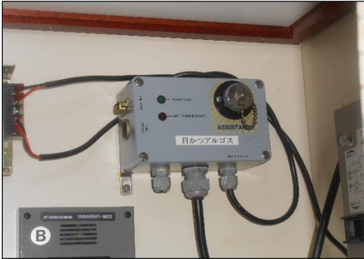
a) VMS during first inspection
